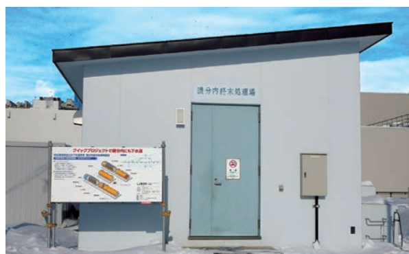
▲磯分内下水終末処理場工事
